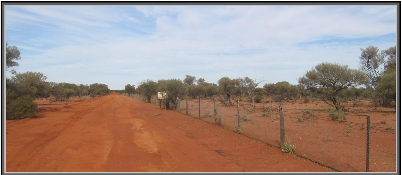
2009 CLEARING & GRADING – BEFORE & AFTER EXAMPLES
